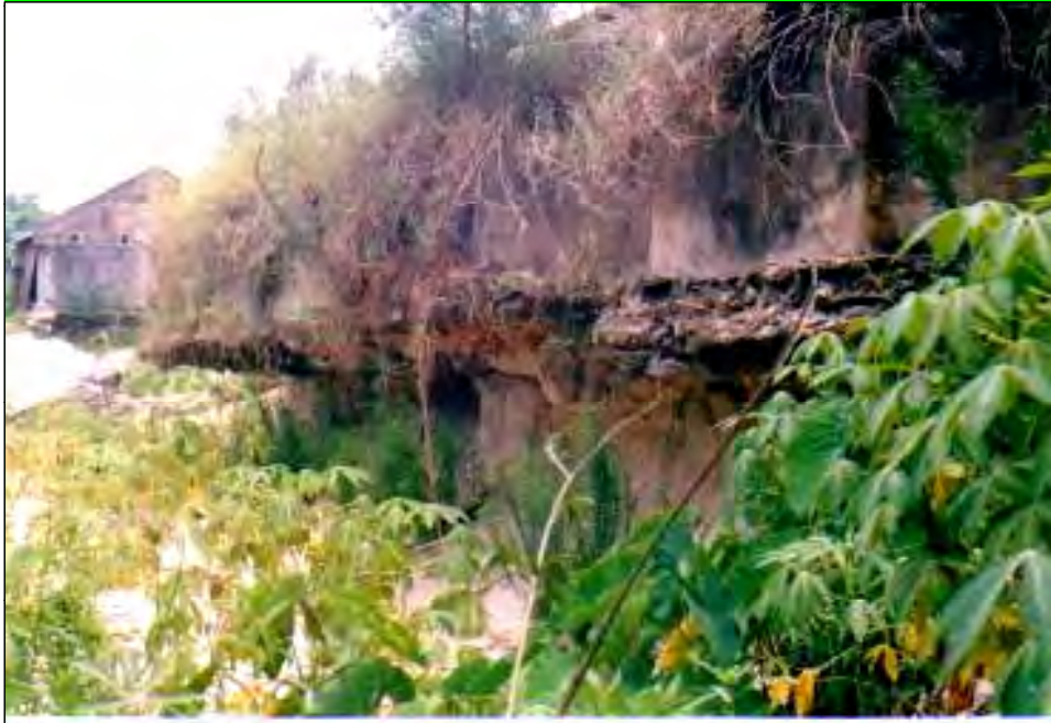
Fig. 13. Sand flow in Le Thuy district (Quang Binh province) in 1999, exposing the pumping station's foundation...
