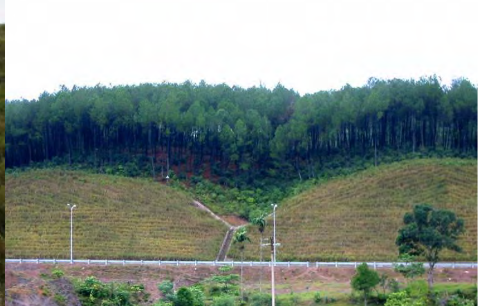
Vetiver protects the cut slope of HCM HW in Quang Binh
