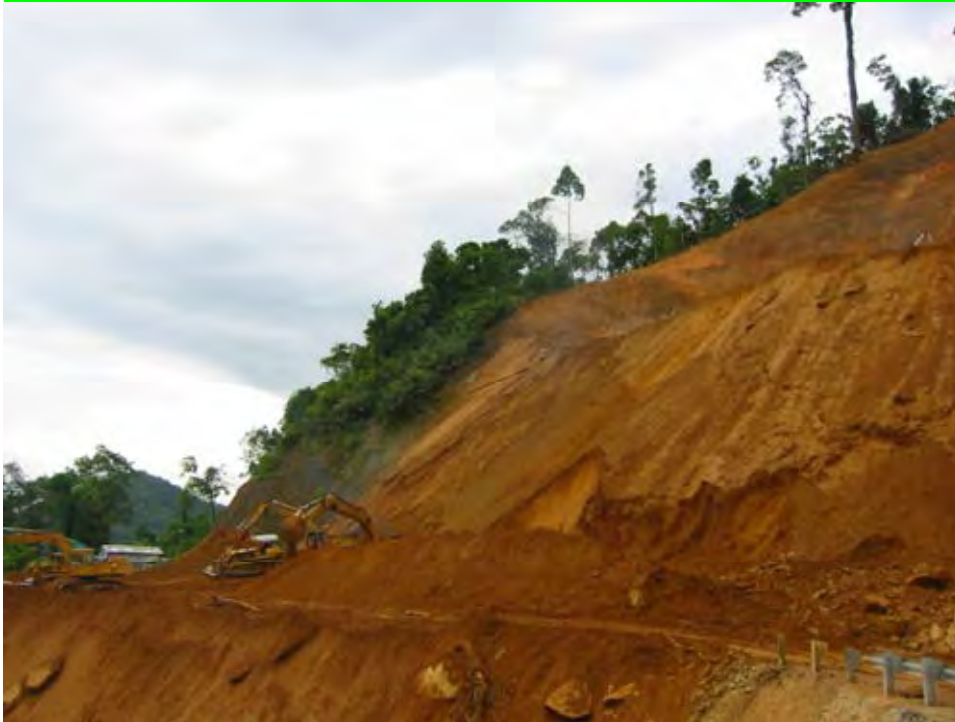
Fig. 7. A big landslide in the completely weathered granite at A Roang Pass, Ho Chi Minh Highway (Thua Thien-Hue province).
