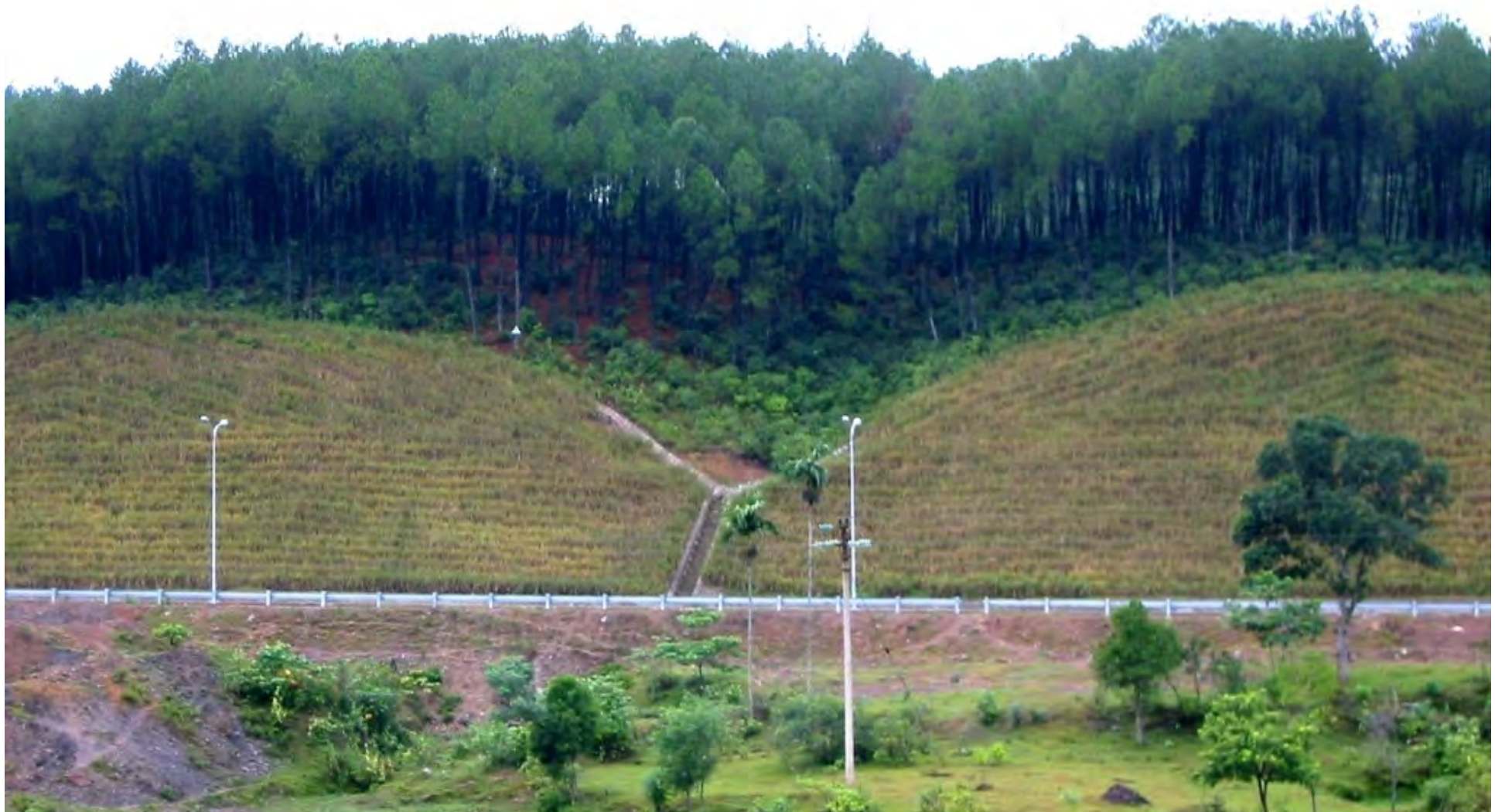
Vetiver protects the cut slope of HCM HW in Quang Binh
