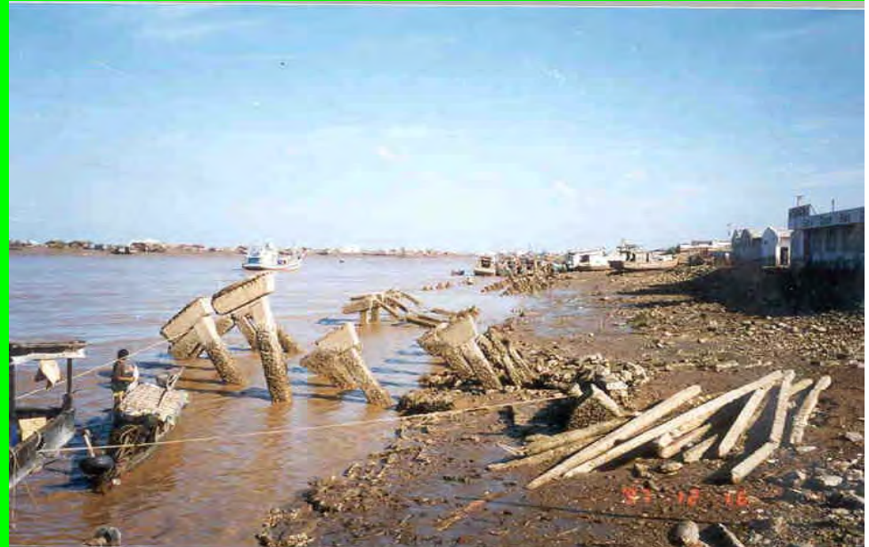
Fig. 6. River bank erosion along Ganh Hao River (Bac Lieu province), causing complete collapse of the fishery jetty.
