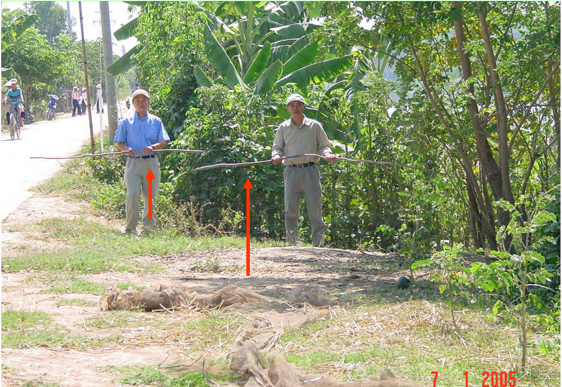
A precious piece of land 5m wide is kept intact due to Vetiver
