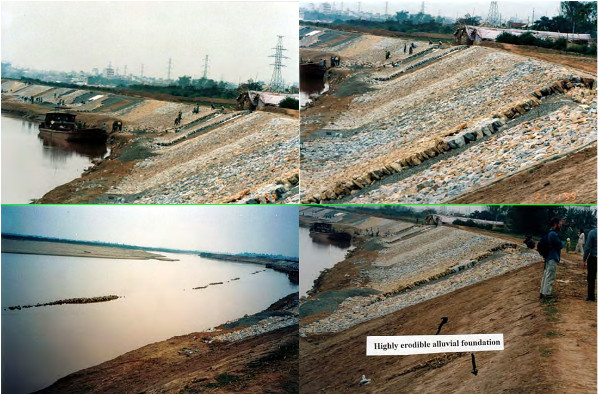
The bank of the Red River in Hanoi is repaired after recent flood using gabions and rock baskets
