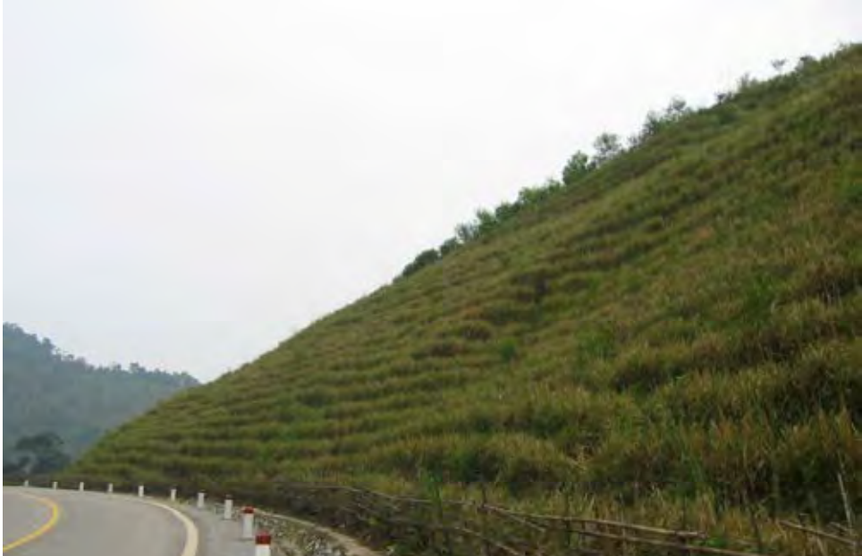
Vetiver protects the cut slope of HCM HW in Quang Binh
